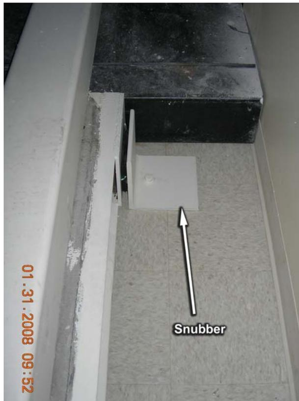
**Figure 12:** Snubber installed at end of inertia base to restrict lateral movement.
