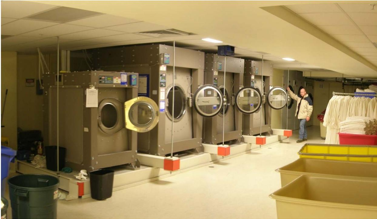
**Figure 13:** Washer/extractors on retrofitted inertia base.
