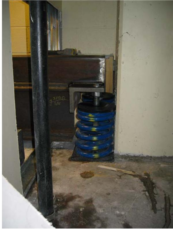
**Figure 10:** Spring isolator at rear of base at column.
