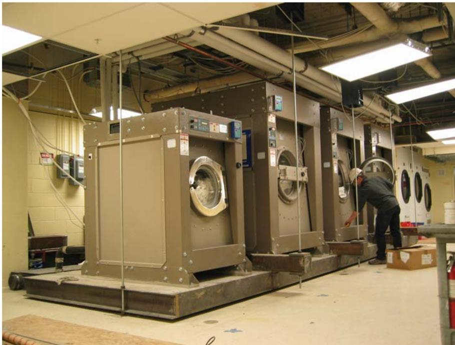
**Figure 11:** Inertia base during installation.
